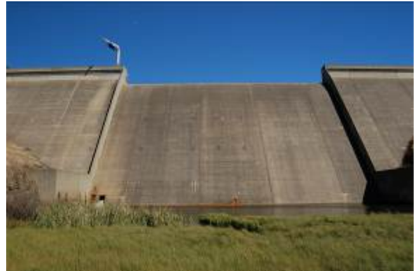
Figure 3. Tantangara Dam on the Murrumbidgee River essentially acts as a large diversion weir and diverts water to the Eucumbene Dam for electricity production (Source: S. Williams).
