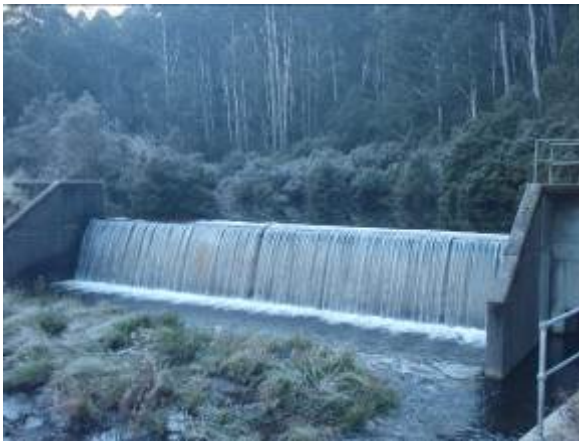
Figure 2. SMRIFs to the Geehi River are delivered via Middle Creek Weir. Water is released by over topping the weir (Source S. Williams).
