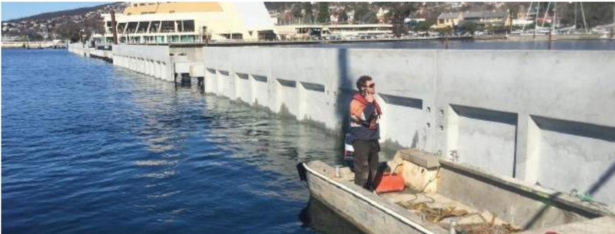
Figure 2. Example of a fixed wave attenuator. Source: Tas Marine Construction.
