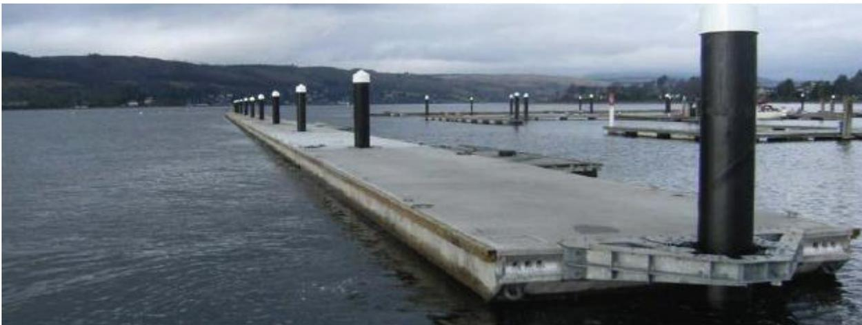
Figure 3. Example of a floating wave attenuator. Source: SF Marina.
