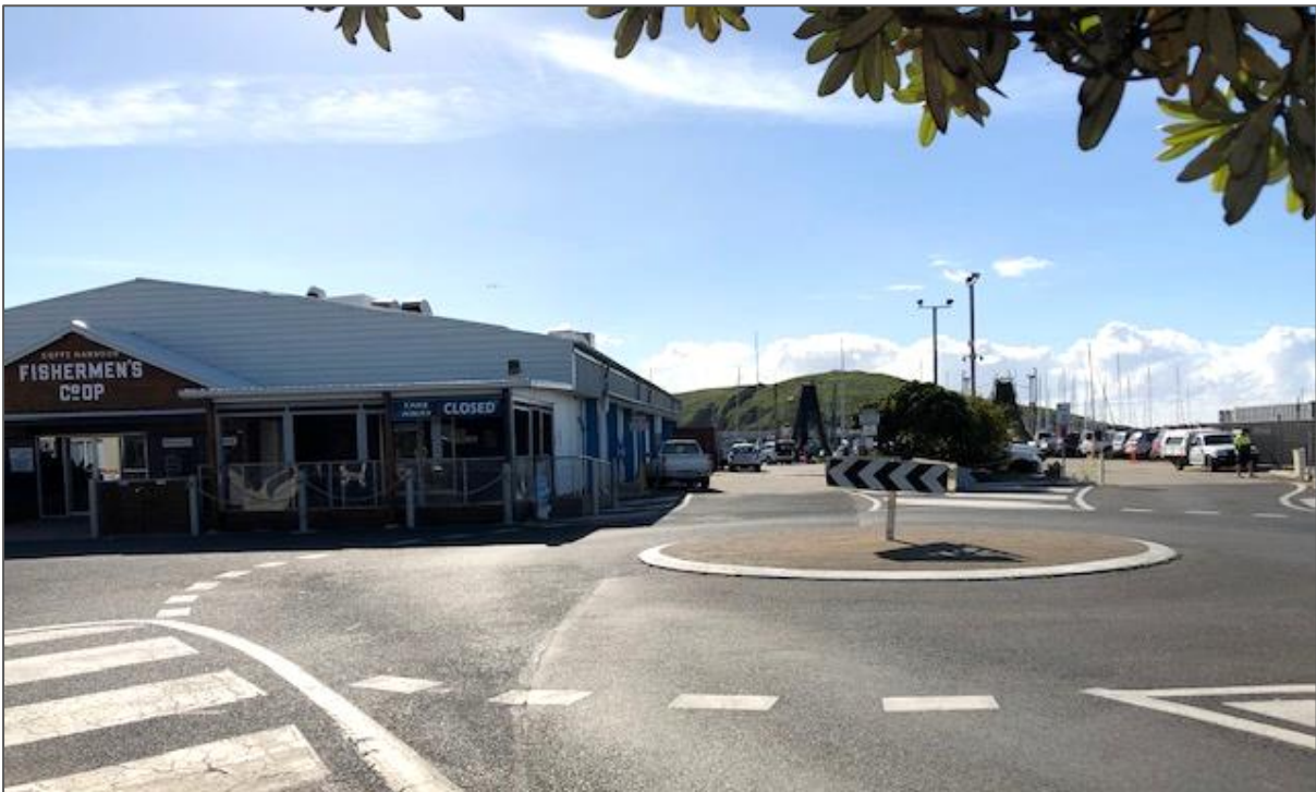
Figure 1 Coffs Harbor Fisherman's Co-op - view from Marina Drive
