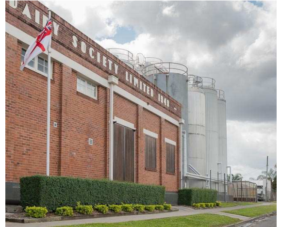
The Richmond Dairies processing plant at Casino, NSW
