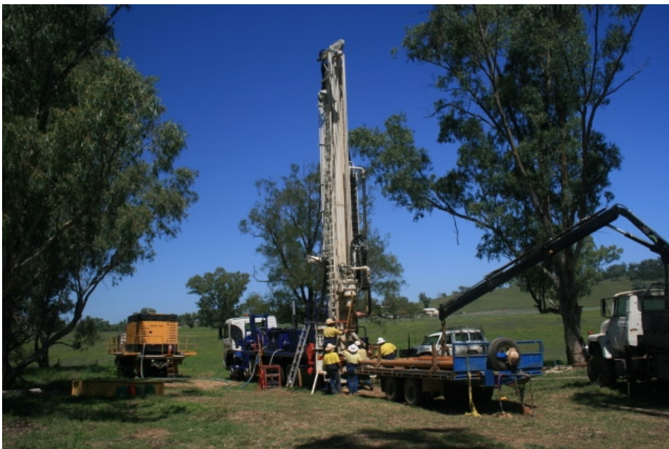
Figure 2: A drill rig similar to this will be used to install the monitoring bores
