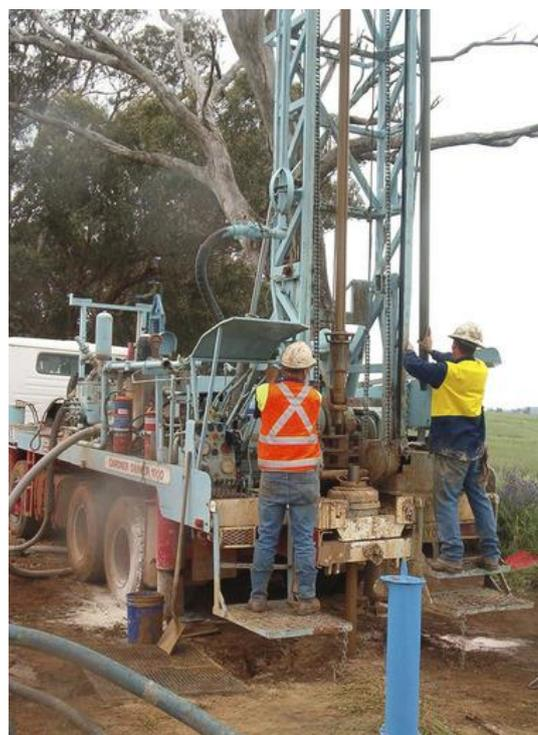
**Figure 1. Licensed groundwater drillers sinking a bore.**
