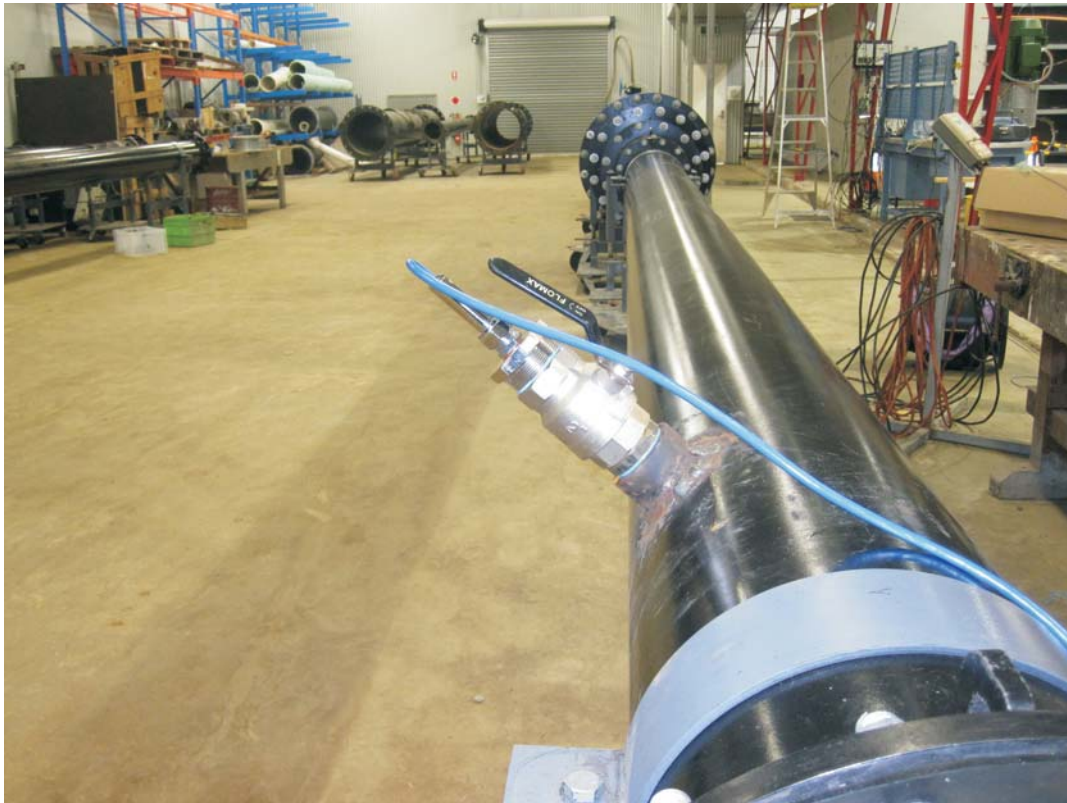
MACE FloPro3 installed in DN300 pipe
