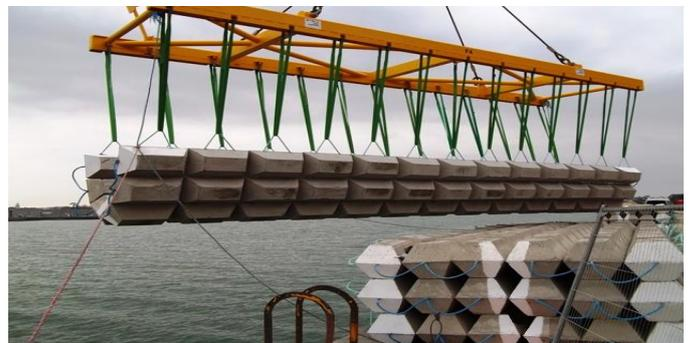
**Typical scour protection being lowered into position**
