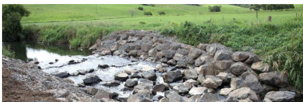
Erosion control works
