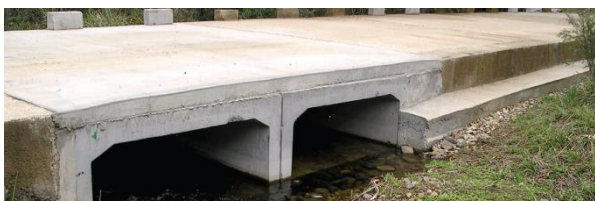
Culvert crossing on a river
